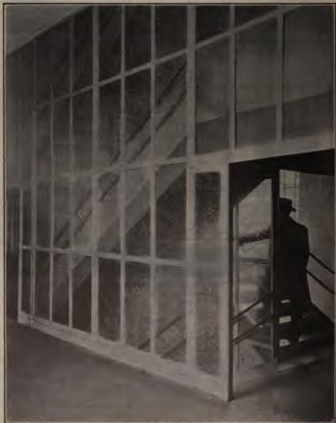
Photographic view of Steel and Wire Glass Stairway. Courtesy of The Mississippi Wire Glass Co.
